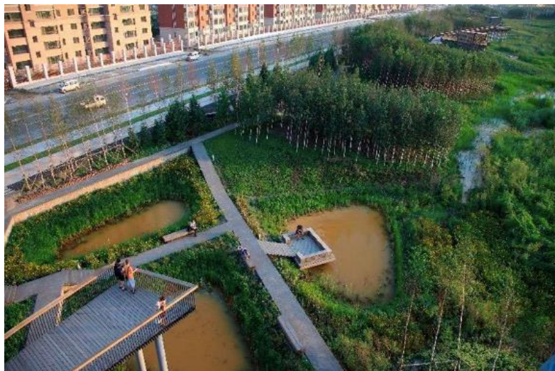
Figure 10: Zhengzhou, one of China’s sponge cities built to manage stormwater run-off and flood damage
